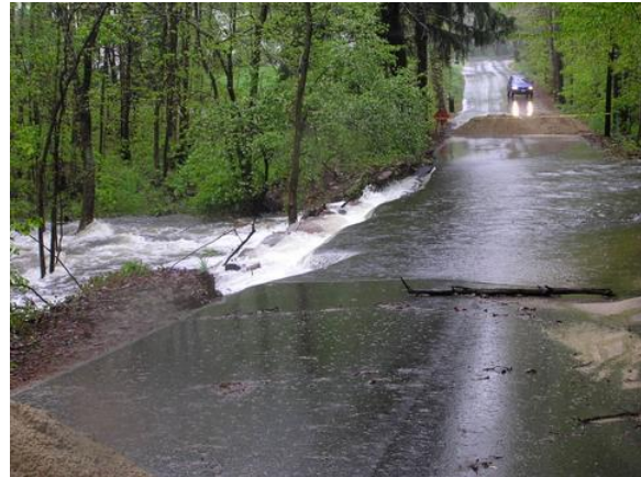
Flooding Along Edwards Mill Road May 2006
