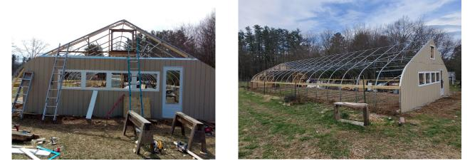
There are a few remaining tasks before the new plastic cover can be applied which will be the final step of the repair work. The care and approach used for these end wall repairs will ensure that any future repair or replacement of the main plastic cover, will be economical and predictable.
